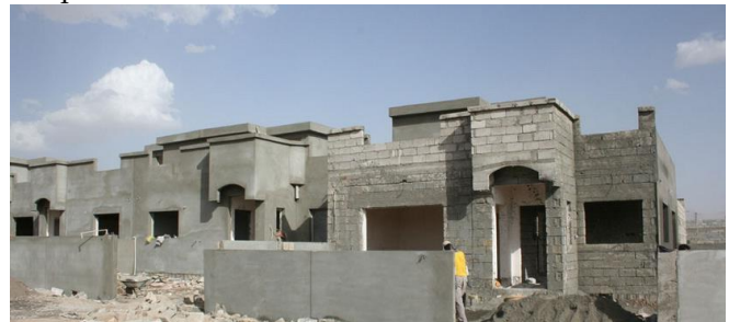
Fig (4) : An example of single-story URM buildings in the KR
